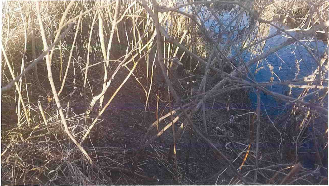
Woody vegetation and erosion near Sta. 4+00 +/-.
