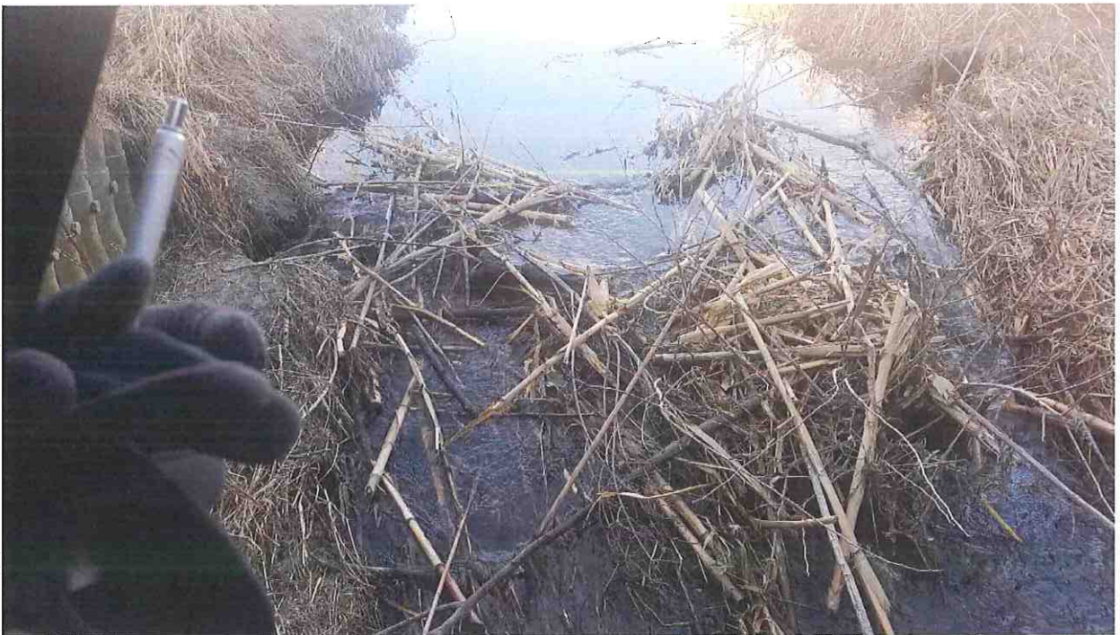
Beaver dam looking west from Sta. 4+00 +/-.
