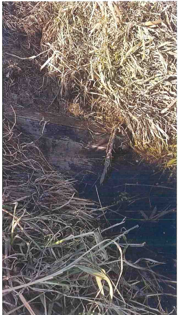
Wooden tile outlets on opposite sides of Open Ditch. Both near collapse and submerged. →
