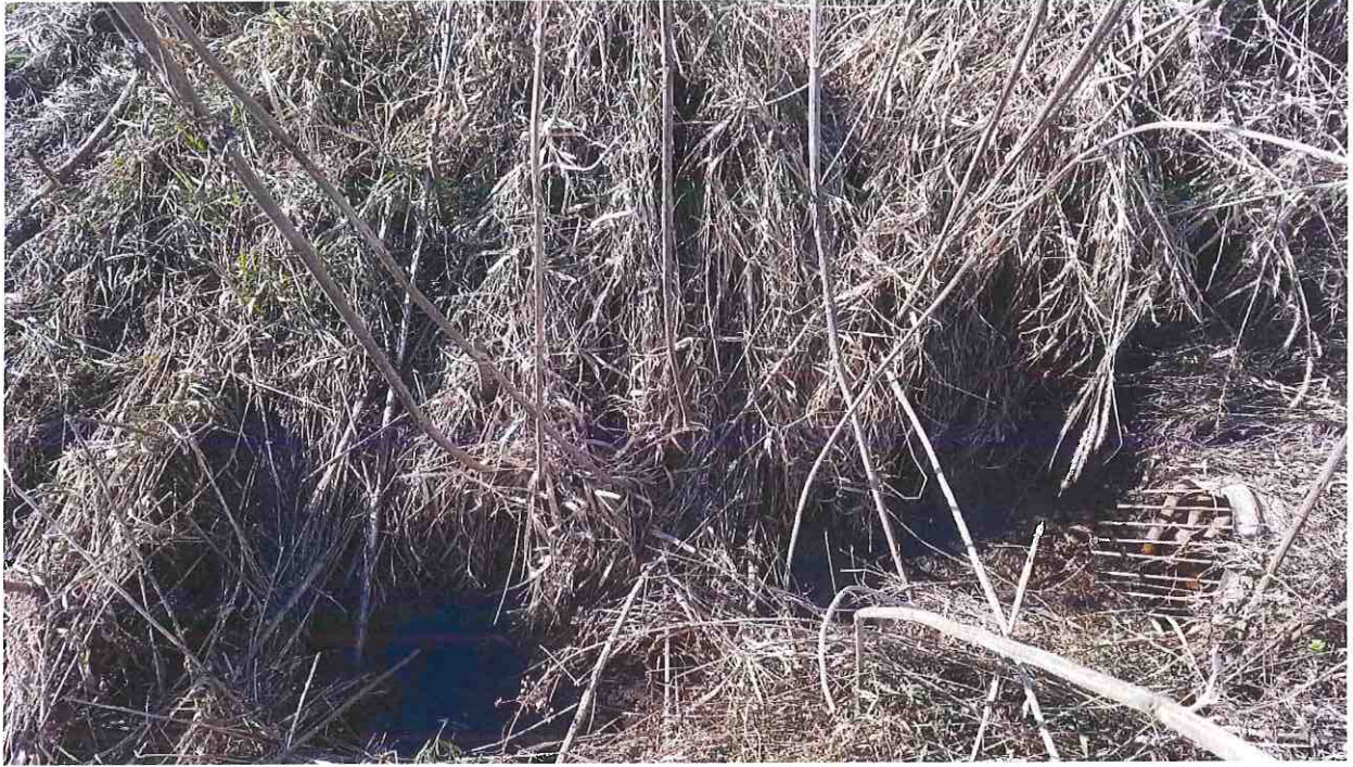
Tile outlet cut 8' into bank.
