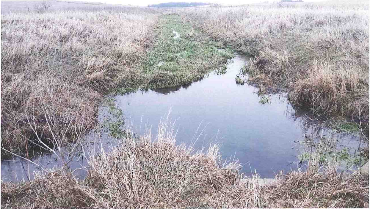
Heavy sedimentation downstream of bulkhead with meandering channel.
