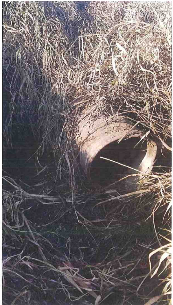
Rusty tile outlet partially crushed, surrounded by heavy erosion, and cut into bank.→
