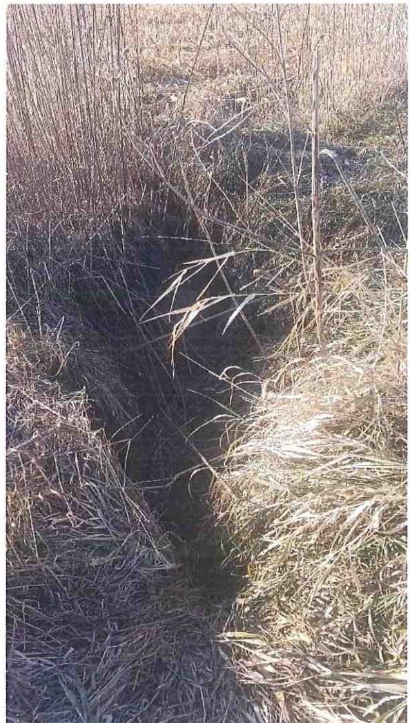
Heavy erosion on the south ditch bank. →
