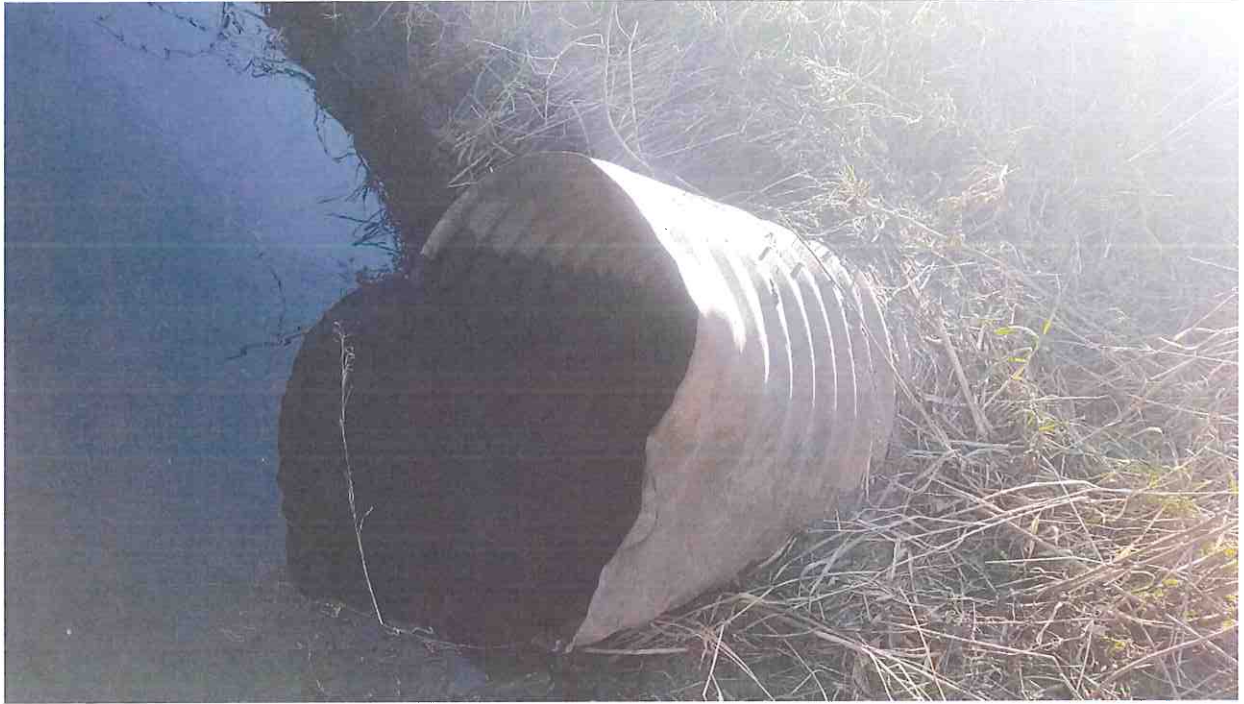
Close-up of above surface drain.
