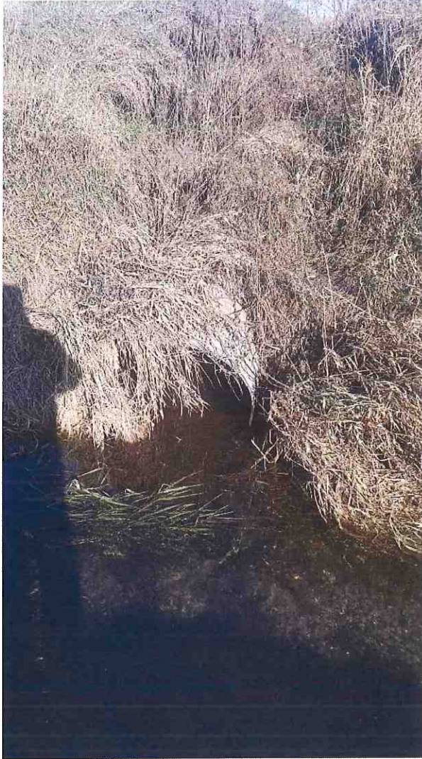
Tile outlet collapsed and buried. Tile is dumping water and cut 30' into bank causing erosion.→
