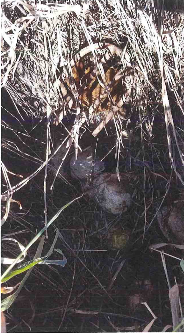
Wooden tile outlet collapsing and cut into bank. →
