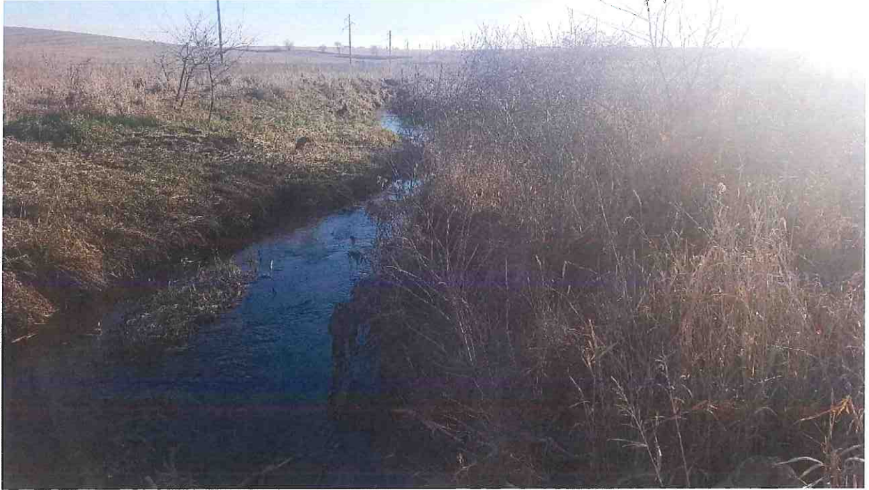
Sedimentation, woody vegetation, and meandering of Open Ditch at Sta. 4+00 +/- looking downstream (both pictures).
