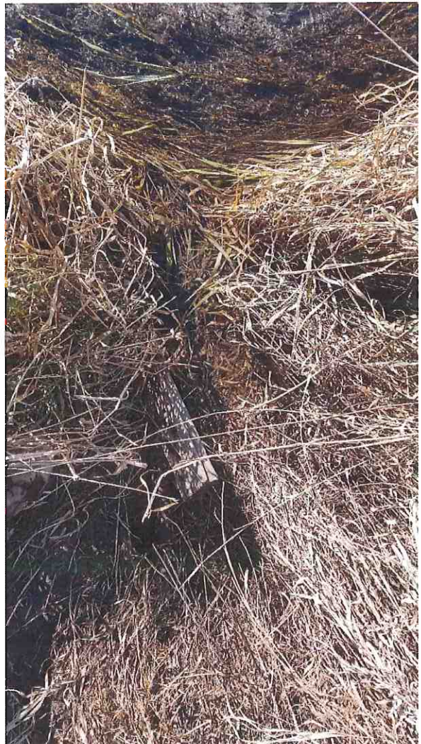
Collapsed and buried wooden tile outlet. →
