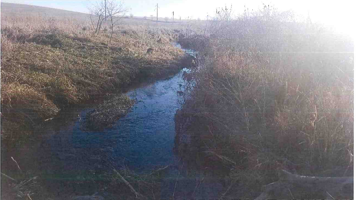
Sedimentation, woody vegetation, and meandering of Open Ditch at Sta. 4+00 +/- looking downstream (both pictures).
