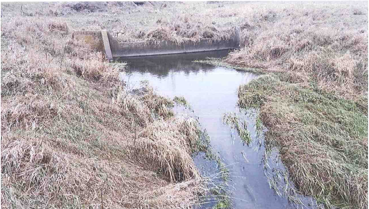
Sedimentation downstream of Main tile outlet.
