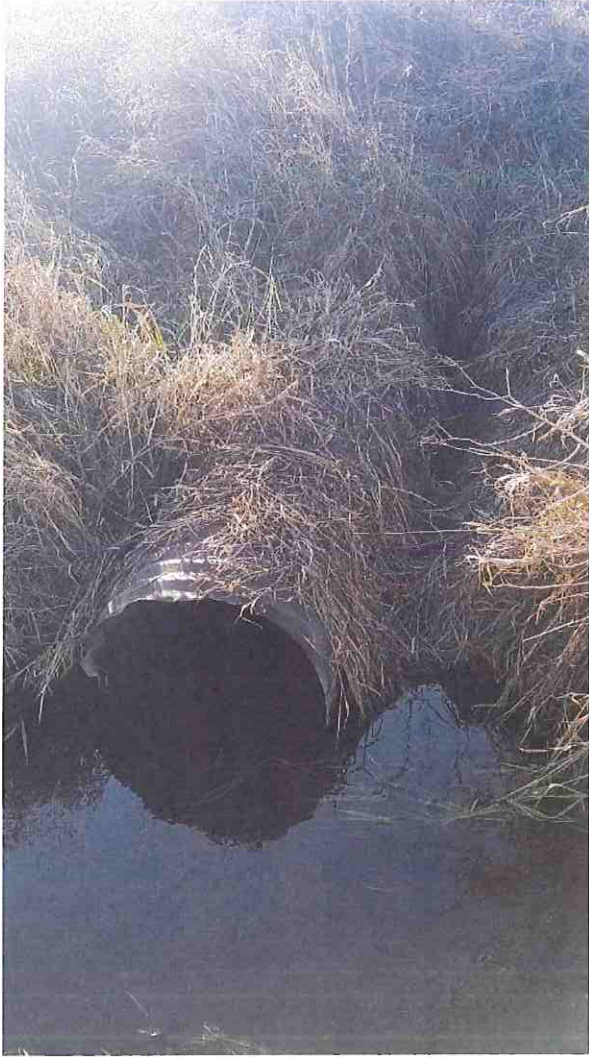
Rusty tile outlet partially crushed, surrounded by heavy erosion, and cut into bank.→
