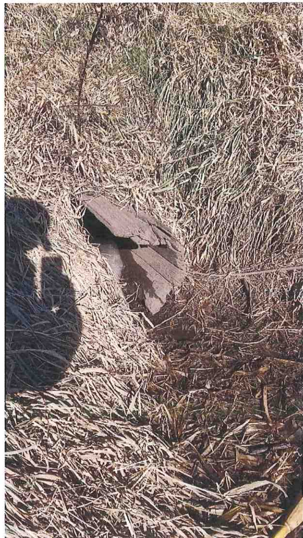
Wooden tile outlet collapsing and cut into bank. →
