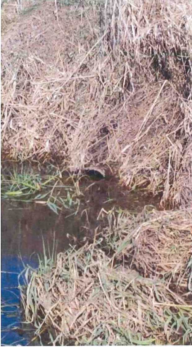
Collapsed and buried wooden tile outlet. →
